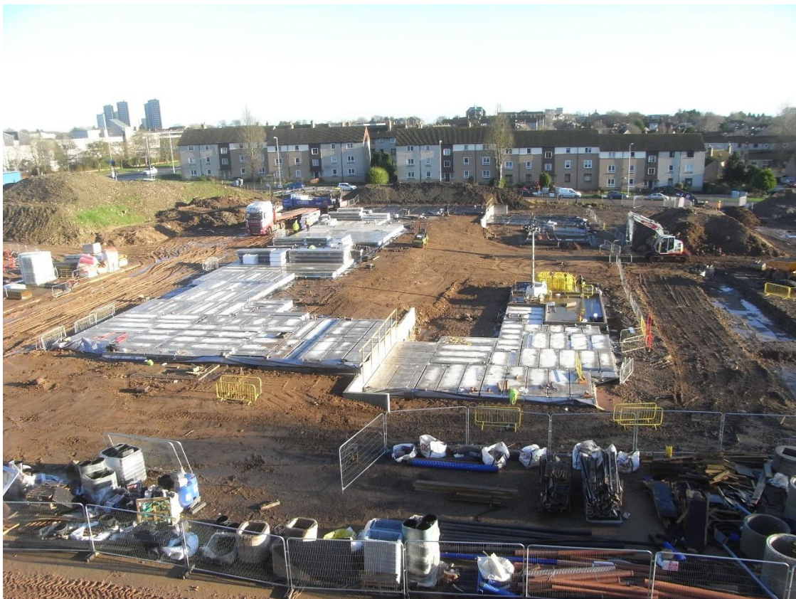
Block 6 – Foundations in Progress (02.12.2020)
