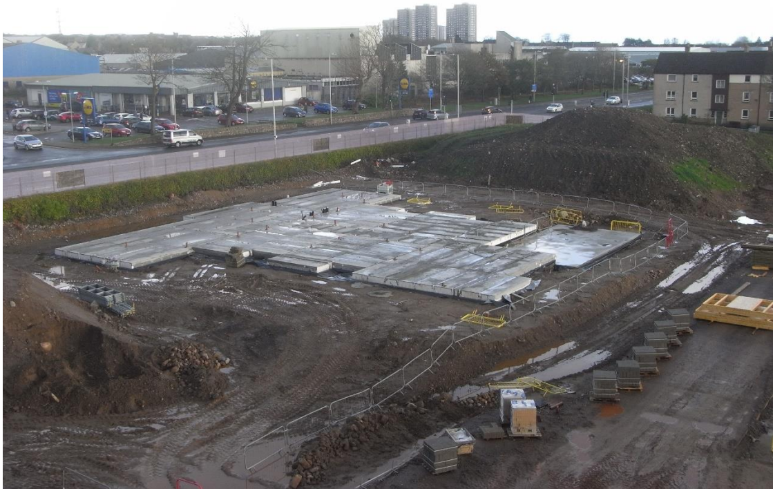
Block 3 – Foundations complete (12.11.2020)
