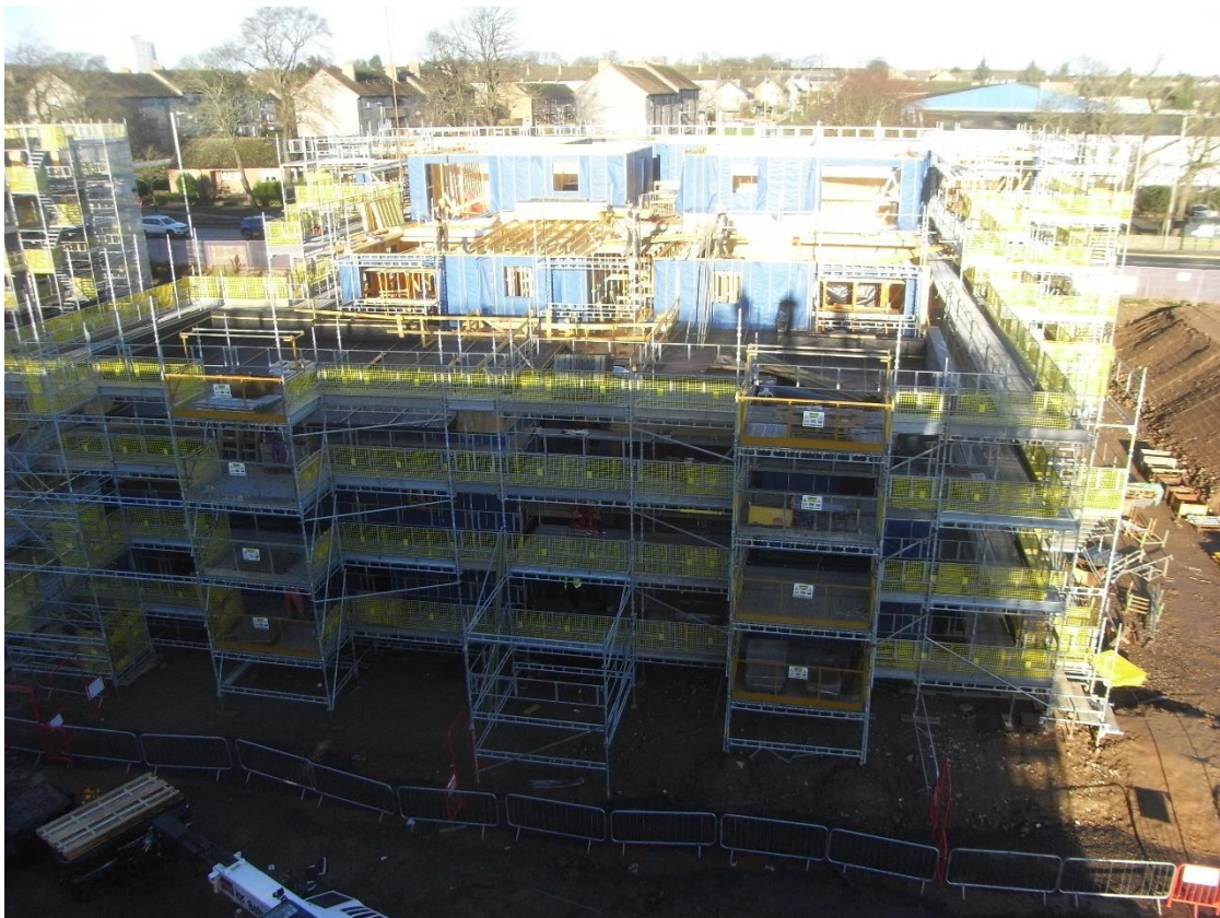
Block 2 – Timber kit erected to top floors; lower roof commenced (02.12.2020)
